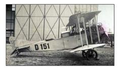
The AEG J II was diverted from the fighter J I and was powered by a 200 hp Benz Bz IV. This biplane was used in huge numbers, together with the LVG C V and C VI. According to John Stroud as many as 71 aircraft were in use, supplemented by AEG G V and Friedrichshafen FF 45 (former G IIIa, twin-engined aircraft). All DLR-aircraft prior to the introduction of the LFR-A (March 1919 and in use
